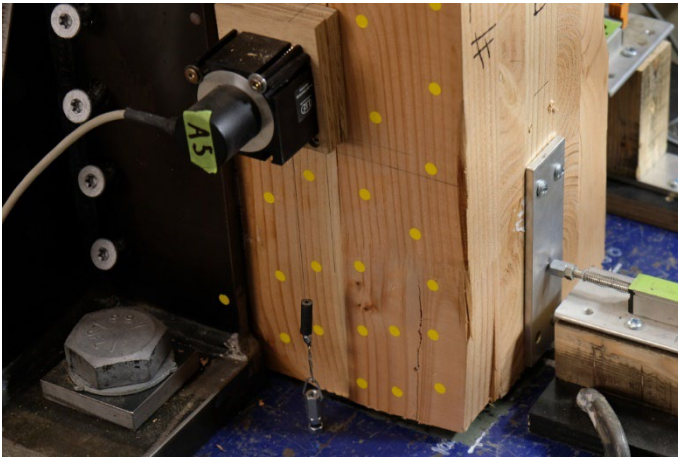
Figure 10: Typical crushing damage observed at CLT wall toe.
